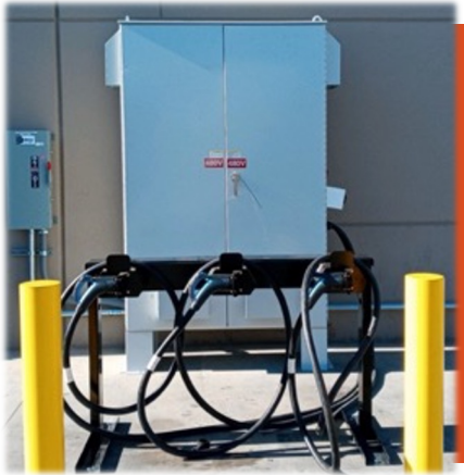
Orange EV Fast Offboard Charging Cabinet: Up to 70 kW
