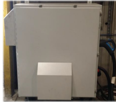
Orange EV Standard Offboard Charging Cabinet: Up to 22 kW
